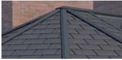
Powder coated aluminium ridge and hip capping is standard
