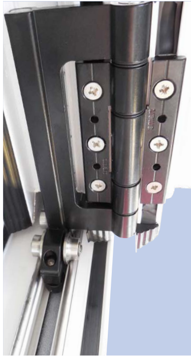
View of retained roller hinge
