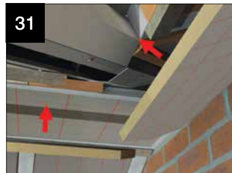
Fit 25mm insulation.
