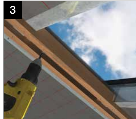
3 IMPORTANT: POSITION CLOAKING PANEL ASSEMBLY IN LINE WITH THE CROSS BATTEN (AS SHOWN) SCREW FIT INTO POSITION.
