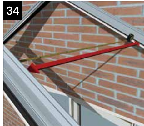
Check that the starter bar and first transom bars are parallel.
