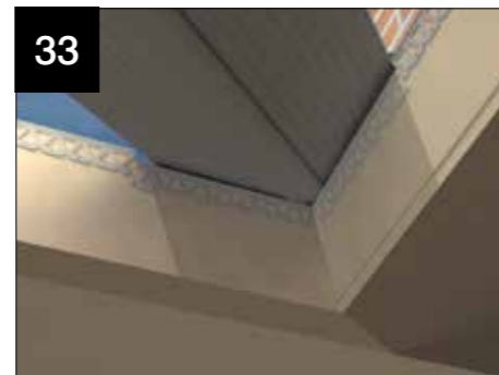
Where plasterboard intersects with the valley undercladding it should be notched to fit and fitted with LVPT250/1 PVCu plasterboard trim.
