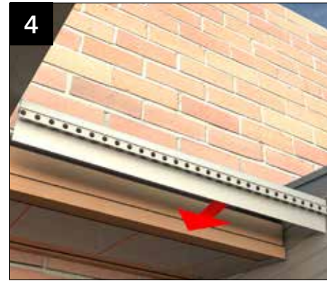
4 Fit LVCT600W and ensure it touches glass. Screw fit using drywall screws) along the lower edge.
