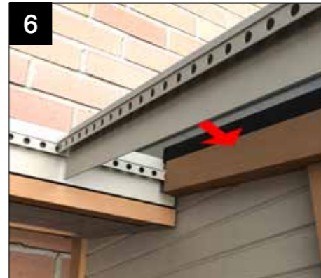
6 Fit LVCT trim - ensure it touches glass. Screw fit.
