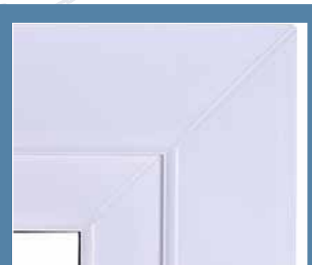
Mitre-welded corners
